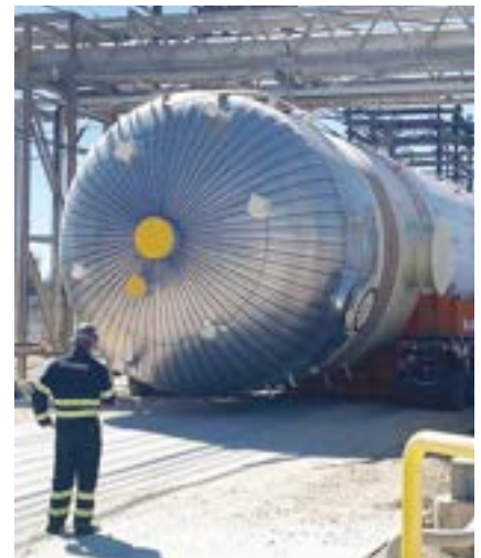
Moving a complex debutanizer that weighs more than 1.2 million pounds from a port to a refinery requires the right transport partner.
