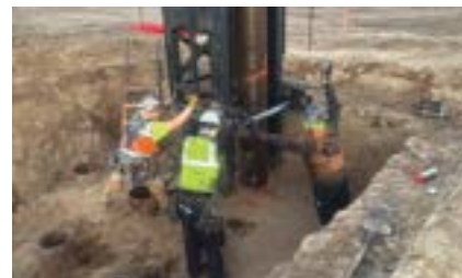
Jarrett Foundations drives a Nucor Skyline 16-in. by 0.500-in. ERW pipe pile to depth.
