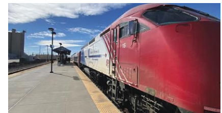
Kimley-Horn helped secure a $691-million core capacity grant to fund nine new segments of double tracking for Utah's FrontRunner Forward Program.
