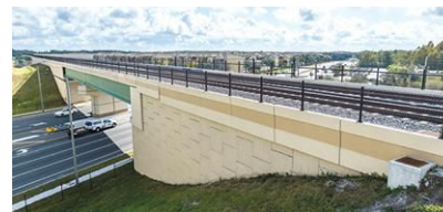
New Reinforced Earth walls were used for bridge abutments and embankments along SR 528 near Orlando International Airport for the Brightline railway project.
