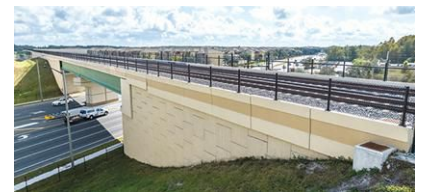
New Reinforced Earth walls were used for bridge abutments and embankments along SR 528 near Orlando International Airport for the Brightline railway project.
