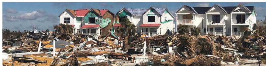
Complicated clean-up continues after Hurricane Michael demolished much of Mexico Beach, Fla.
