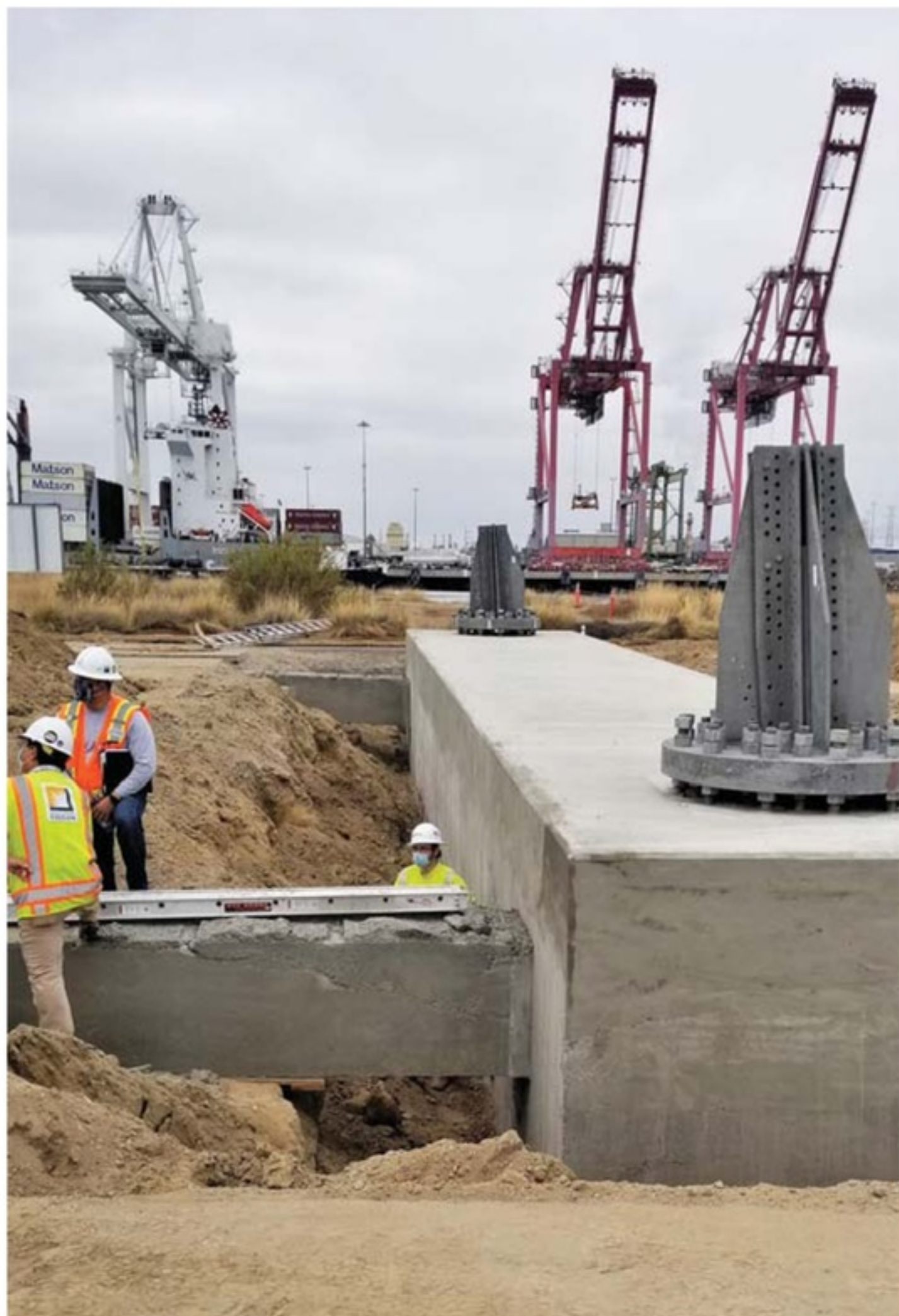
Large grade- and tie-beam system at southern tower.
