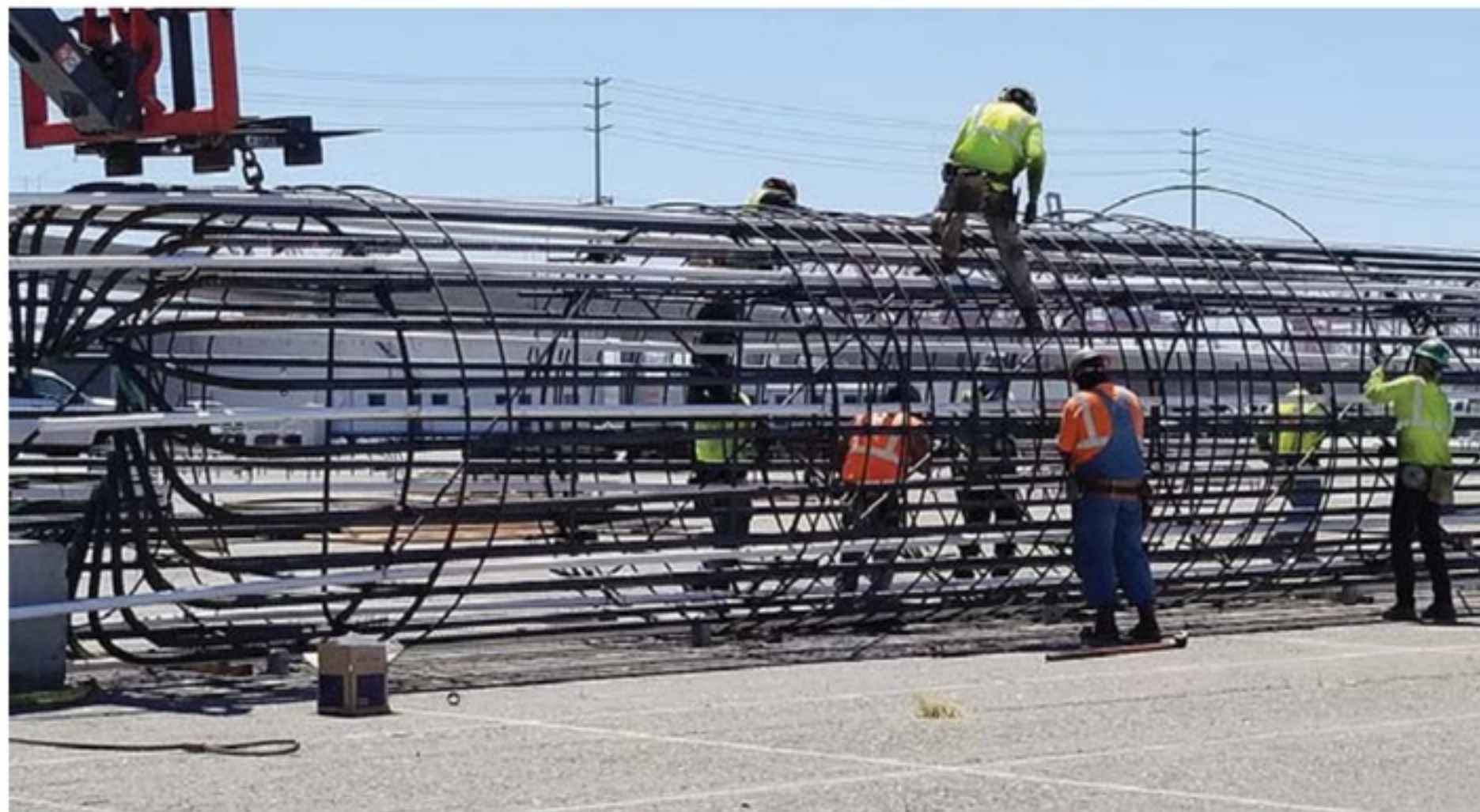
Rebar cage assembly.
