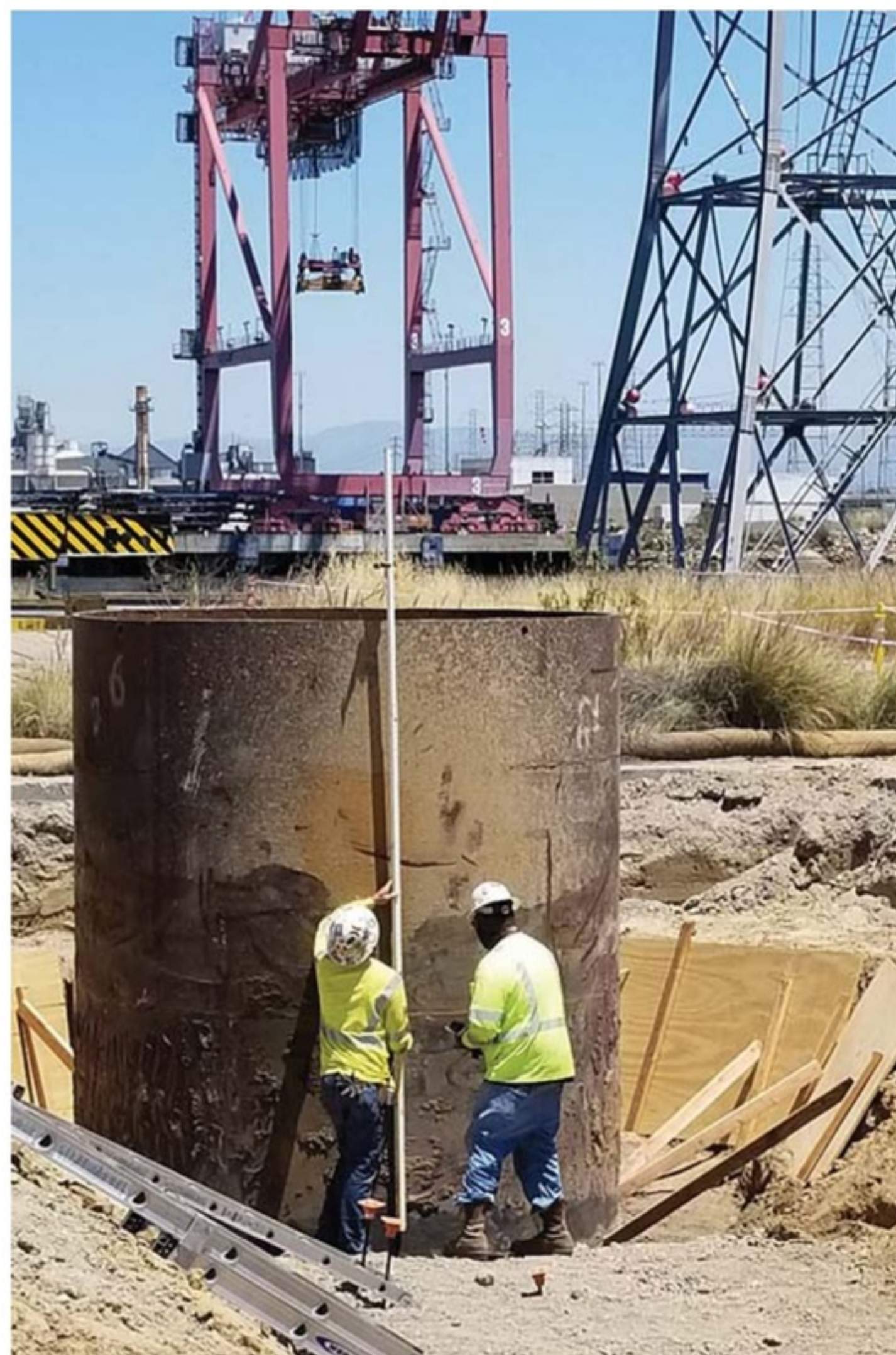
Leg for tie and grade beams.
